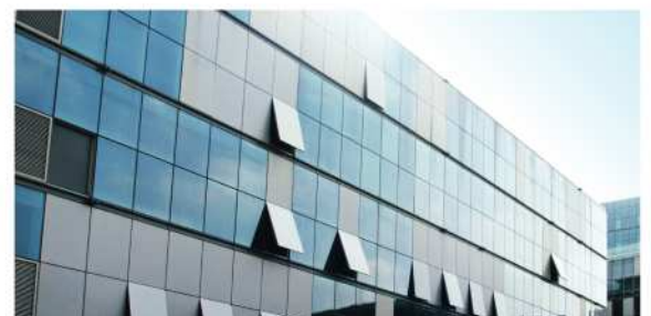
Exterior Wall Construction (Chameleon)
