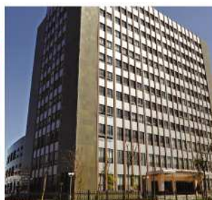
Exterior Curtain Wall Construction(granite)
